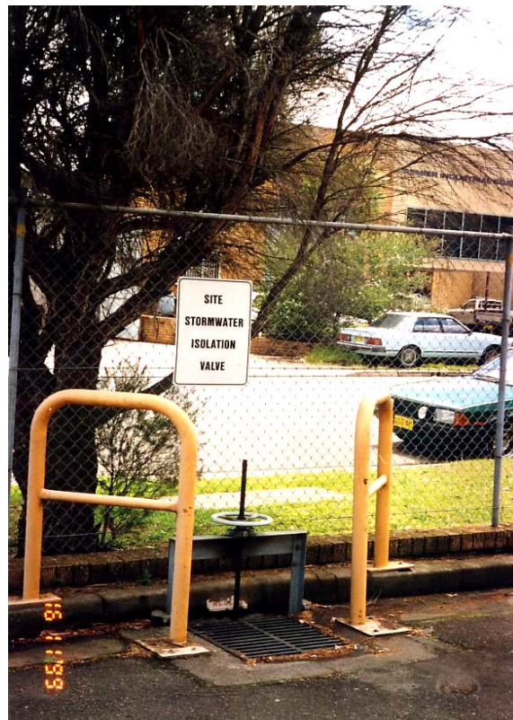
▪ Figure 3 – Location of any Stormwater Isolation Valve.
