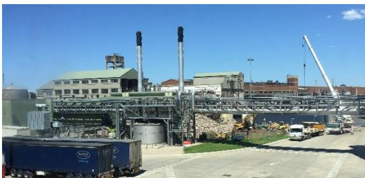
Figure 2: Pre-B5 demolition and SWT installation
