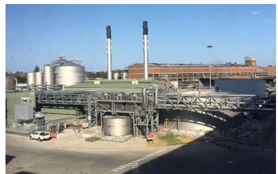
Figure 3: SWT plant installed
